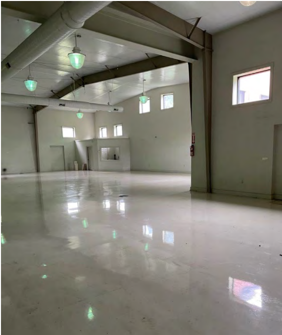
Front section, looking to back, right side section
