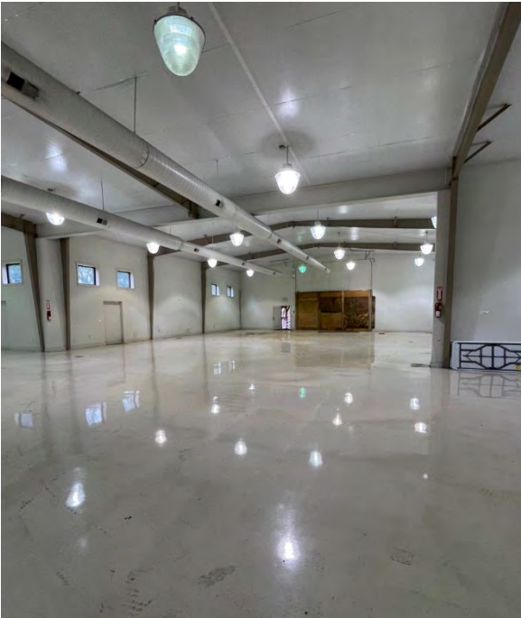
Front section, looking at front of building
