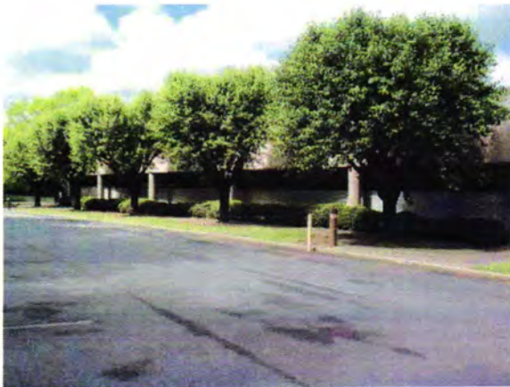
1. FRONT VIEW (EAST)
